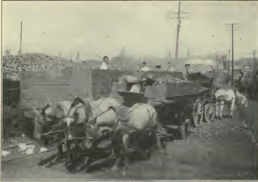
FIG. 41. STORED MATERIALS, A SOURCE OF DUST. View, showing the handling of coal by hand. Many cars of coal are unloaded daily on the team tracks and in the coal yards of Chicago. The dust arising from such operations is caught up by the wind and distributed over wide areas.
